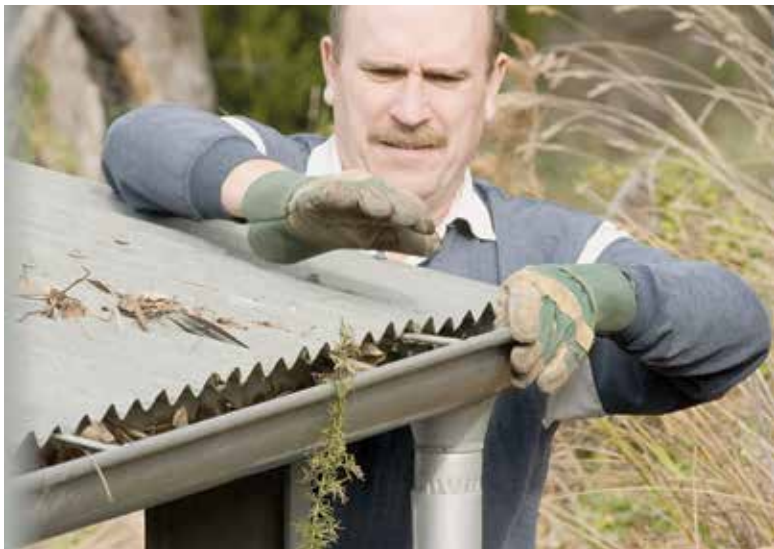
Clear gutters of flammable material
