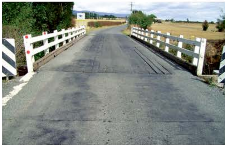
Existing bridge on Pitts Lane.
