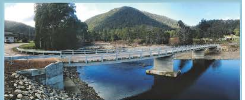
Above: The new Liena Bridge (photo courtesy of TasSpan)
