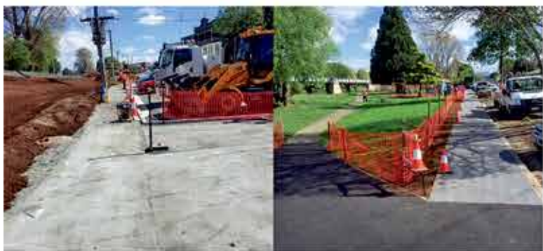
Above: Access improvements underway on West Parade in Deloraine
