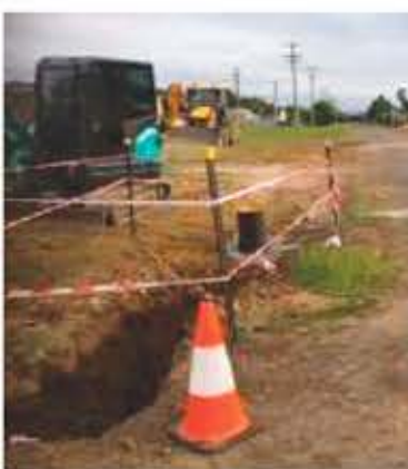
Above: Work in progress along Henrietta Street in Bracknell
