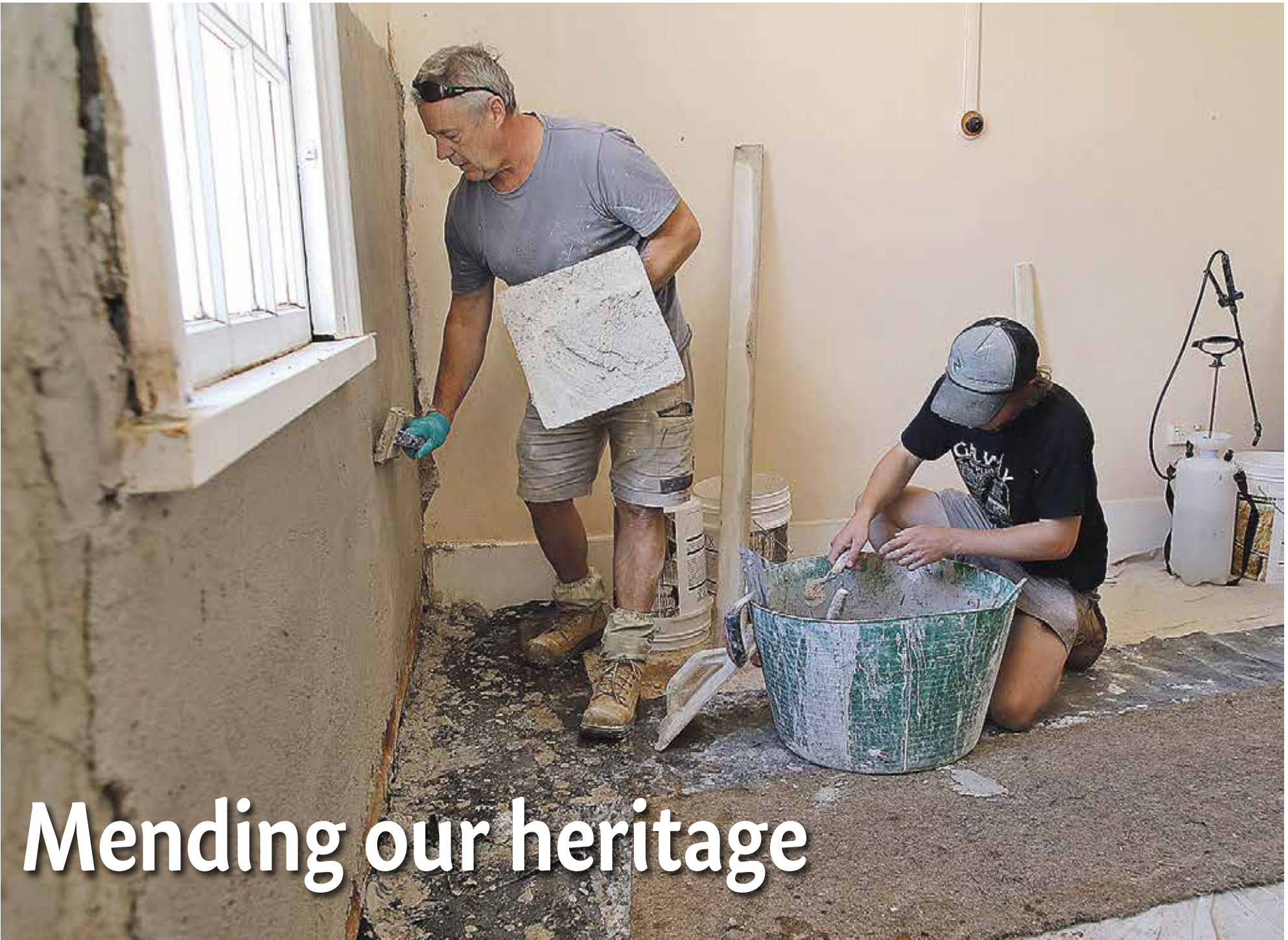
Dave Conway of Launceston, expertly applying new lime mortar to the inner walls of the Folk Museum, assisted by Ben Earle.
