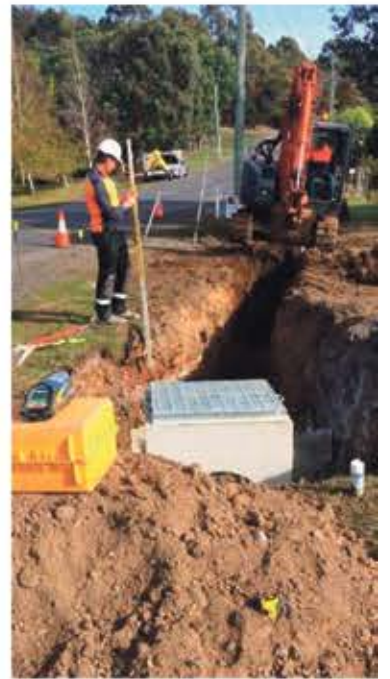
Above: Footpath construction in Blackstone Heights will improve pedestrian connectivity.
