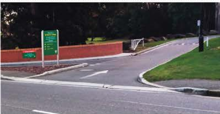
Above: School pick-up and drop-off times will be made easier with upgrades proposed for Mount Leslie Road, adjacent to St Patrick's College.
