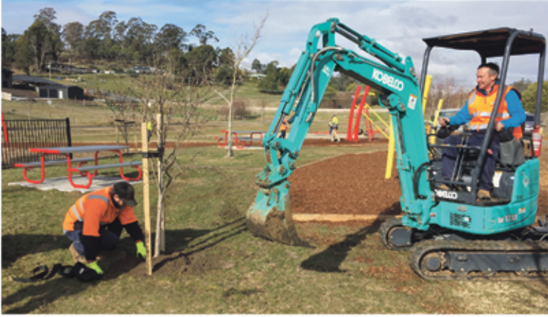
Above: Council's Works Crew completes tree planting at Blackstone Park
