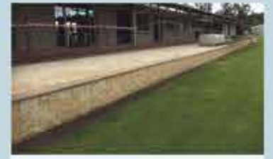
Retaining Wall Extension & Additional Paving Prospect Vale Park, Prospect Vale
