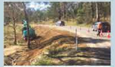
Road Shoulder Widening Pateena Road, Travellers Rest
