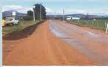
Road Reconstruction Osmaston Road, Westbury
