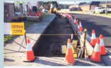
Parking Bay Construction Winifred Jane Crescent, Hadspen
