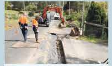
Footpath Construction Blackstone Road, Blackstone Heights
