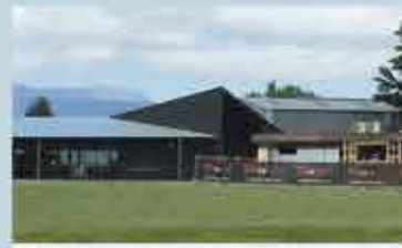
Sports Pavilion Upgrade Westbury Recreation Ground, Westbury
