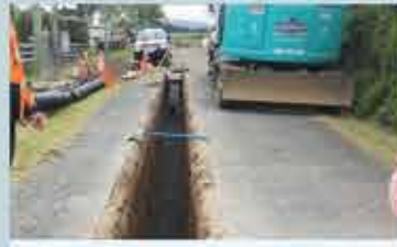
New Storm Water Infrastructure Meander Valley Road, Westbury
