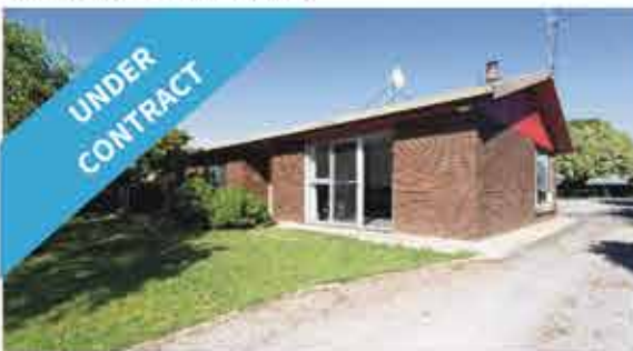
16 Caveside Road MOLE CREEK
